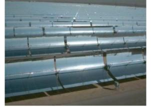
A Parabolic Trough Power Plant
